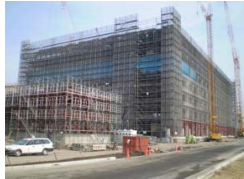
(Construction status in the beginning of Nov.)
